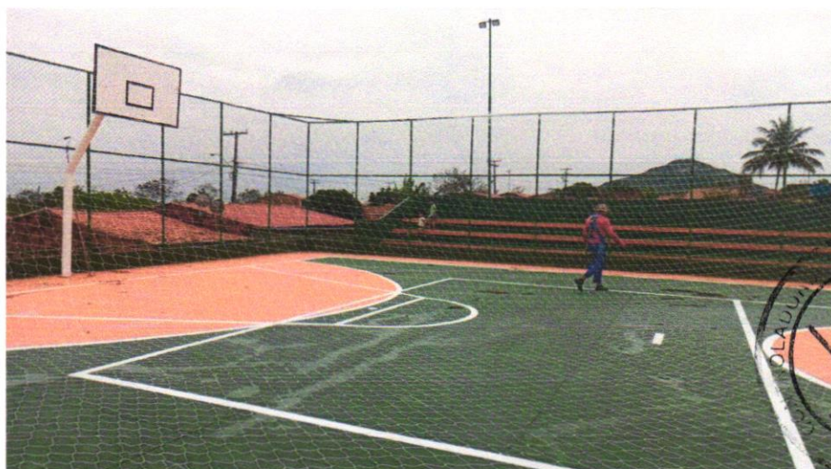
Foto 06 - Tela de nylon, fio 30-36 (3,6mm), malha 10x10cm
